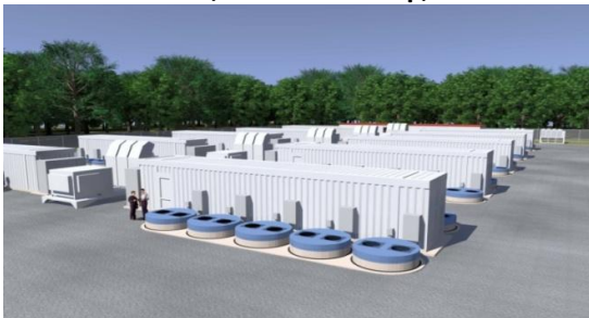
20 MW, Hazle Township, PA
