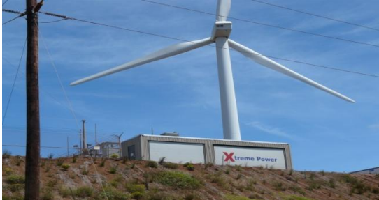
Xtreme Power KWP 1
